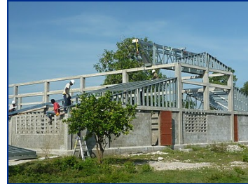
Under Construction Nov. 2011
