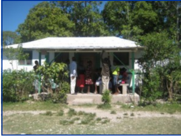
The Former Klinik Espwa
