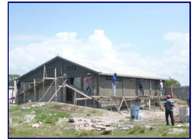
New Restrooms Under Construction
