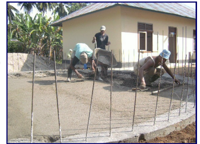
Dome Home Construction
