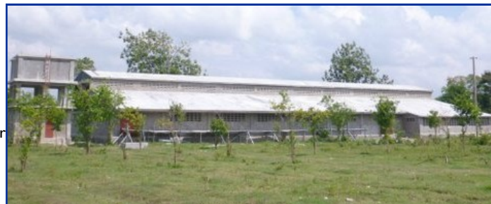
Photo Right: Side view of kitchen and dining hall. Water tower on the left end.
