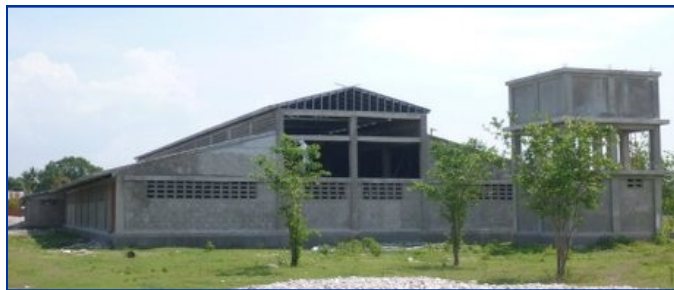
Photo Left: Kitchen end view near well tower for water access
