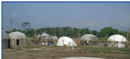
Dome Homes in Various Stages of Construction
